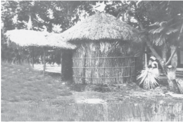
Fig. 4.2 Many poor families live in kutchas houses
